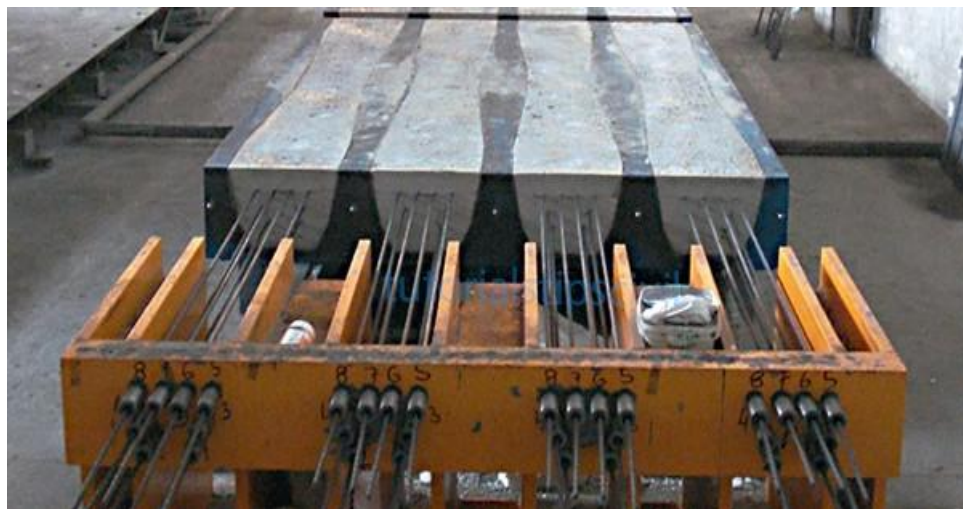
Figure 1.3: Pre-tensioning Concrete
