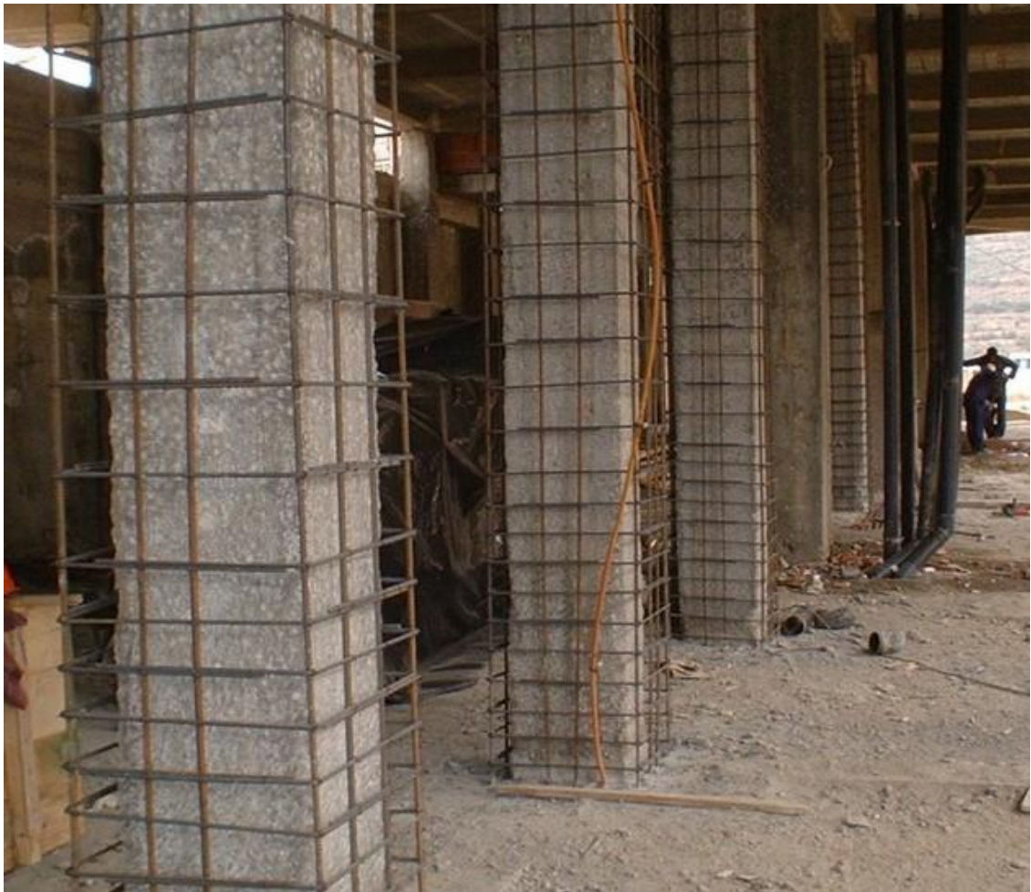
Figure 1.8: Concrete Jacketing (Source: https://sslaxmienterprise.com/?page_id=662 )
