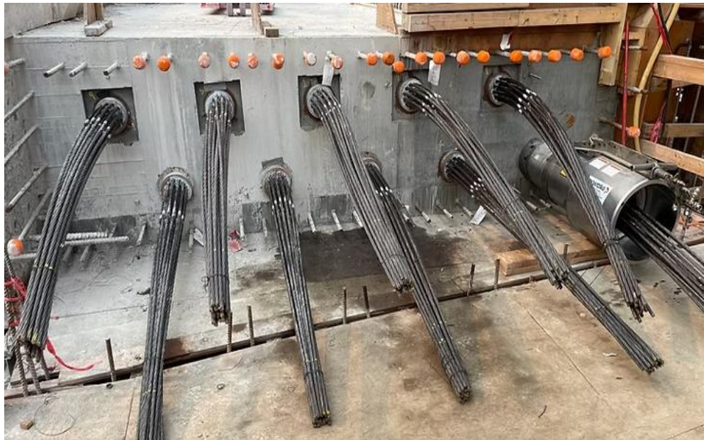
Figure 1.4: Post-tensioning Prestressed Concrete
