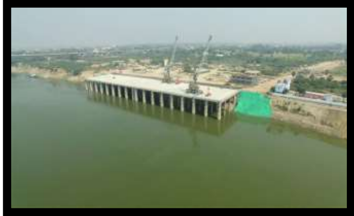
(Fig.no. 17 View of IWT Multimodal Terminal Varanasi)
