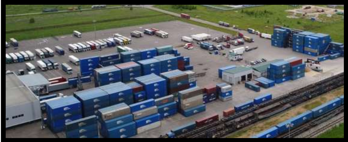
(Fig. No.28. Model Plan for development of Freight Village at Varanasi, Source of Image: www.google.com dt.05.04.2018) 22
