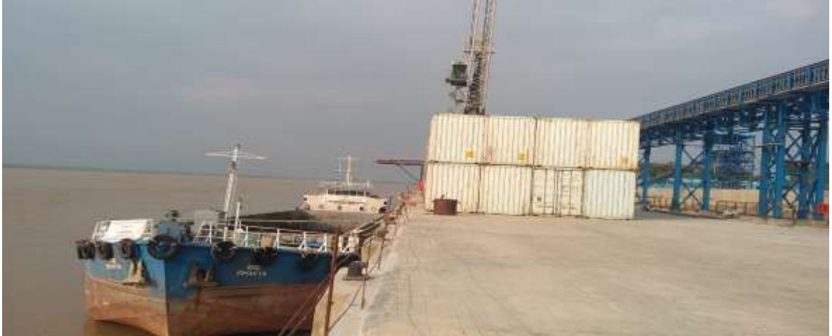
(Fig.No.186. Container unloading at MMT Sahibganj, along NW-1)
