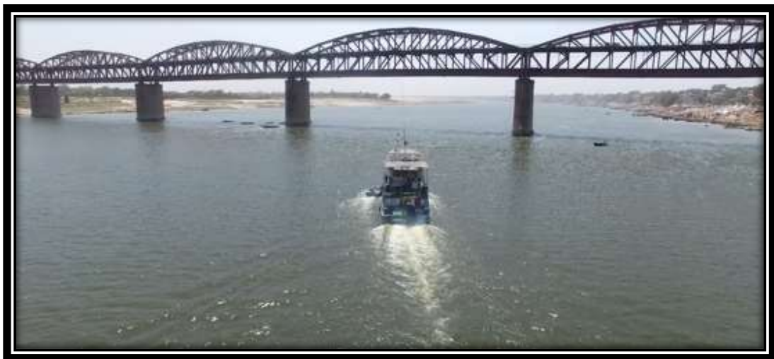
(Fig. No 196: IWT Survey Vessel Navigating near Raj Ghat Bridge at Varanasi)
