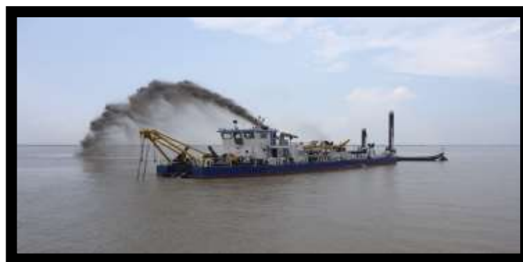
(Fig. No.13. View of dredging operation in Progress along NW-1)
