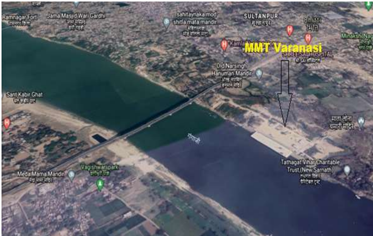
(Fig.83. Google Earth Satellite View of Multi Model Terminal at Ramnagar, Varanasi)
