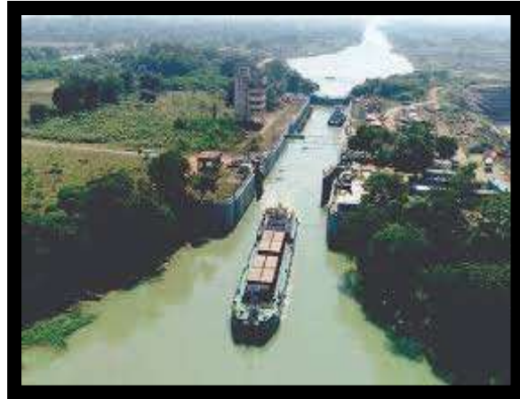
(Fig. No.20. View of Old Navigational Lock Gate, Farakka, source: IWAI official Tweet on 29.11.2.19) 19
