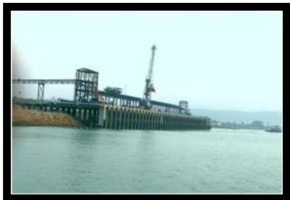
(Fig.No.18. View of IWT Multimodal Terminal Sahibganj)
