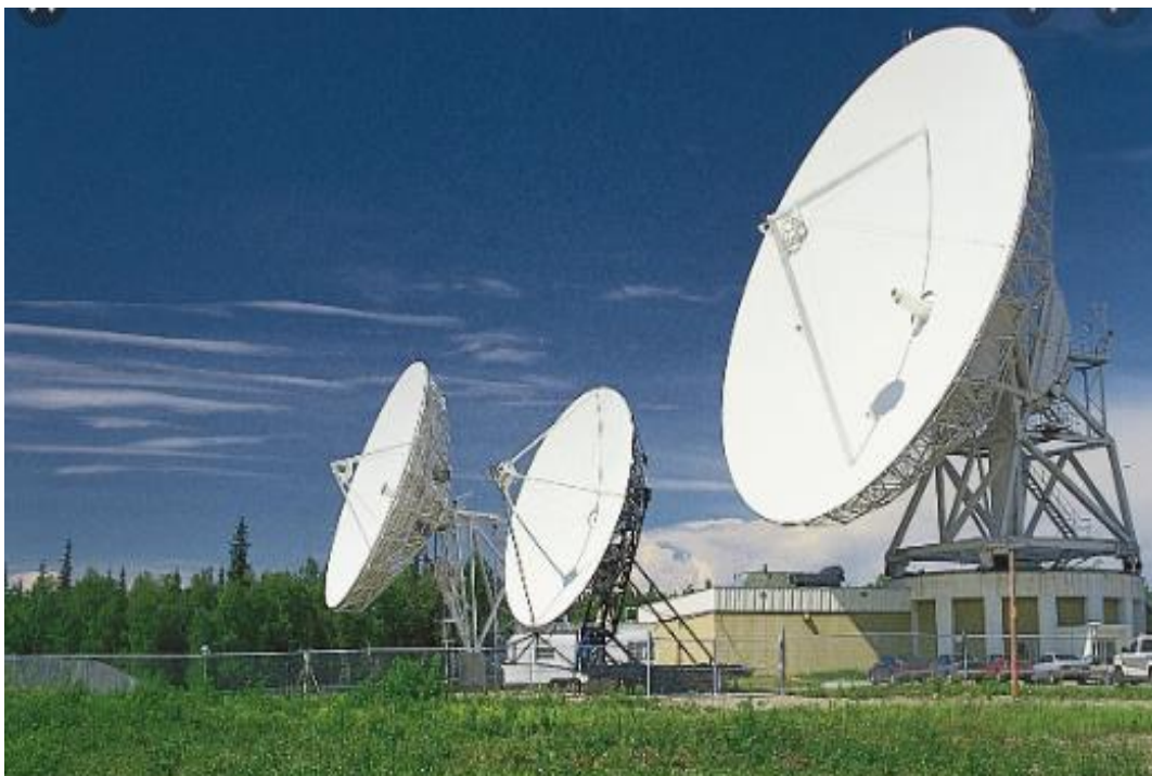
Figure 1.13:Satellite communication antennas
