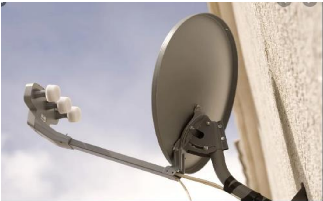
Figure 1.17:Dish antenna with three LNV
